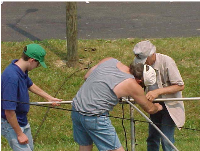
Here Jason KC8LIN and Jeff, KC8KIX and Perry assemble the HF beam antenna for the Phone Station
