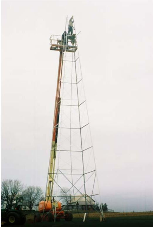
The "Great K8KIP Tower Project" . The bucket truck can be seen in the background helping with the installation. Jim WA8GXM is on top of the tower finishing up the antenna installation.
