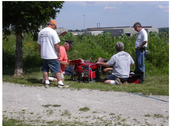
Oh Oh! Murphy was with us on this Field Day. Just after getting going on Field Day, the generator quits running. Carl, Don Igor, Terry & Jim (behind the generator, on the ground) work to get it going. Finally figuring out the trouble the generator was up & running & purring along like a kitten in no time.
