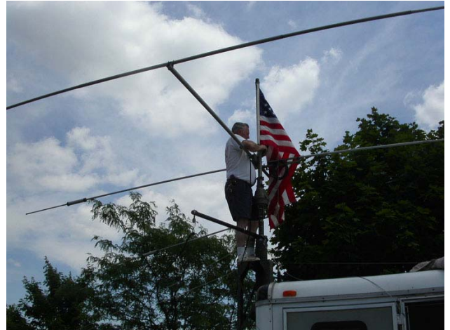
Now it's Jim's turn to finish the installation of the 3 element beam antenna for the phone station on the E-Com
