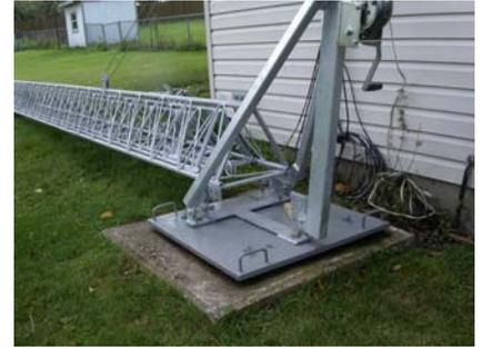
The new tower arrives and is installed to the mount. Also installed is the tilt over mechanism called "raising fixture"
