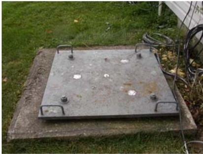
Start with base plate. 1" thick steel, 3' square with a 4'x4'x 5' deep concrete base. You can see where old tower stood as light spots on the base.
