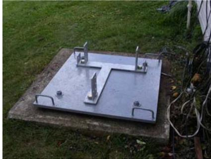
Same base repainted with the new T base/ tilt over mount installed. Holes for 1" anchor bolts had to be drilled & tapped.
